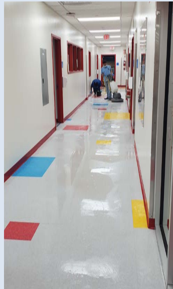
Washington Yu Ying Summer Project Stripping and Finishing Floors
