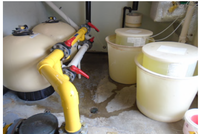
Reserve provides for pool filters, water supply/return piping, chemical treatment equipment and other system components.
