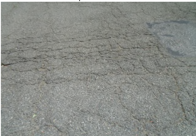
Asphalt pavements have reached the end of their life, they are scheduled to be milled and overlaid over the next 3-years. See our recommendations in comments section to maximize pavement useful life.
