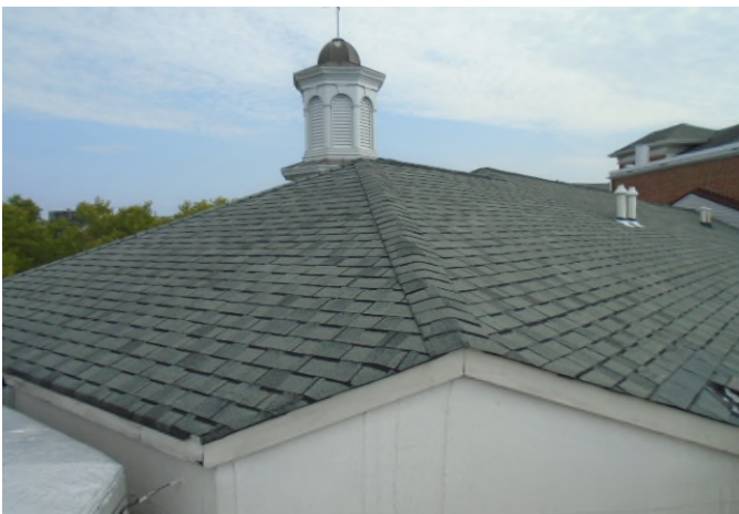
Roofing is shingles with a flat platform for HVAC equipment. There is also a minor amount of standing seam metal roofing.
