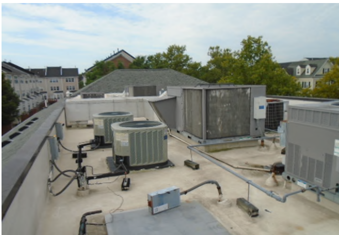
Roof-top mechanical platform. Two older 8 and 3 ton units are scheduled to be replaced. Units are being replaced as needed to maintain building temperature.
