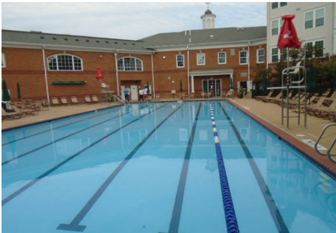
Pools need whitecoating about every five years. Although we allow for this work to occur on that schedule, decision to whitecoat should be evaluated when pools are drained.
