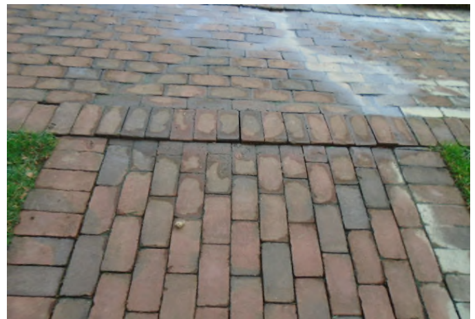
Funding to maintain and repair the brick paver walkways are a reserve component. Settling, heaving, cracks and other defects need to be repaired to maintain a level walking surface.
