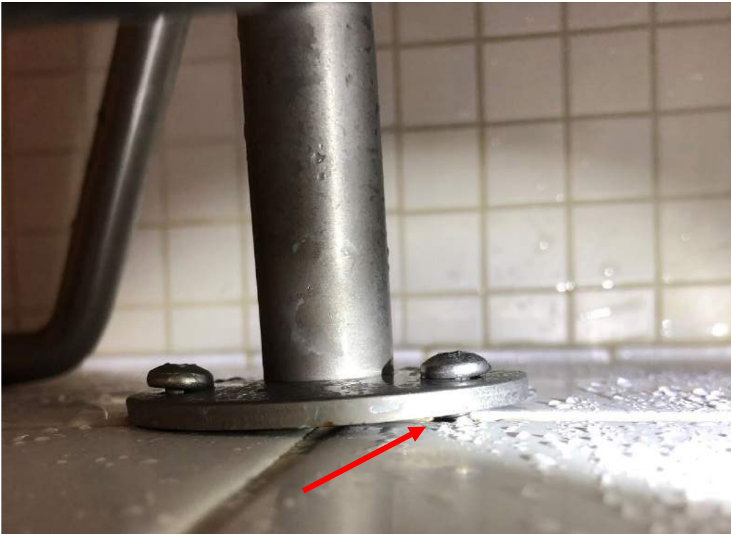
Photograph 8 – Penetration through shower wall. Fasteners were not sealed.
