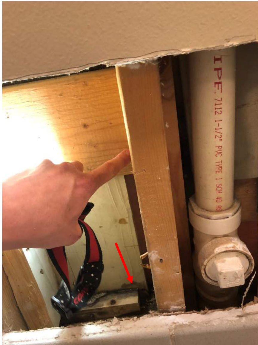
Photograph 7 – Water dripping within the wall cavity at Location A. Note wet spot (red arrow).
