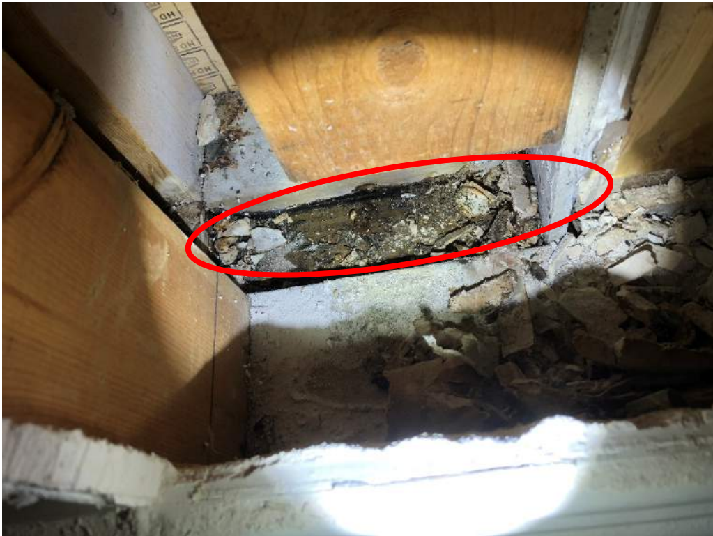
Photograph 10 – Water entering wall cavity beneath bottom plate of wall at end of hallway.
