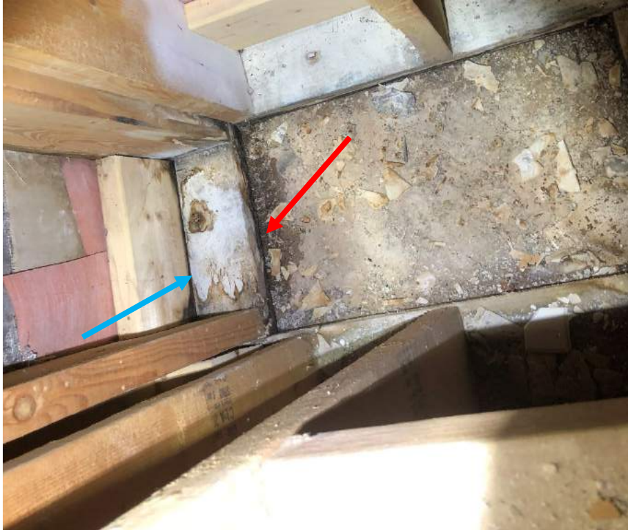
Photograph 12 – Stained wood (blue arrow) and water (red arrow) within wall cavity of men's bathroom. (See Photograph 11)
