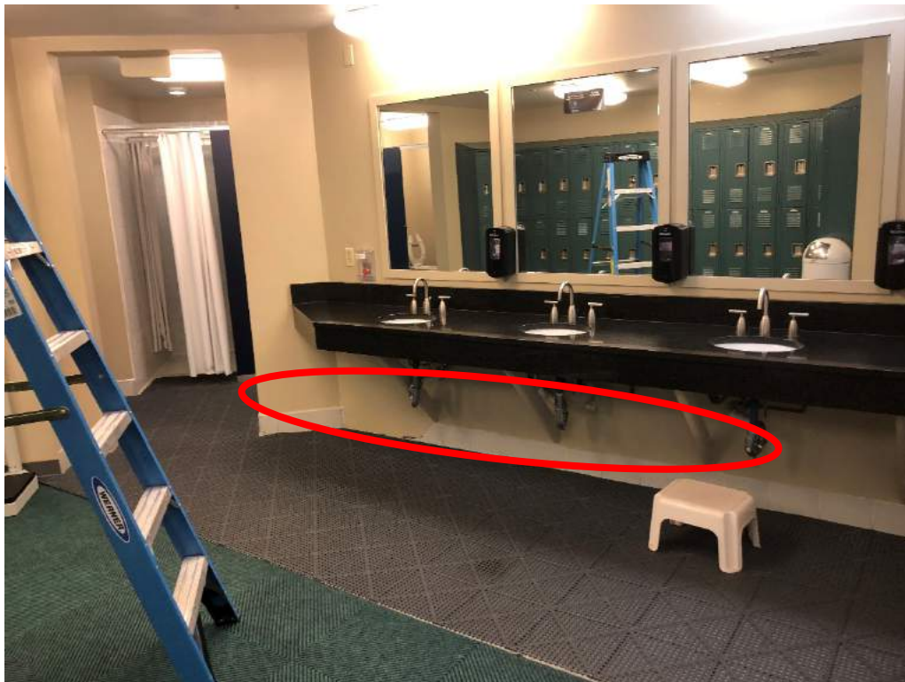
Photograph 2 – Area of previously observed moisture near sinks in men's locker room. This area also includes back side of wall (not pictured). Both areas has a moisture content of less than .2%
