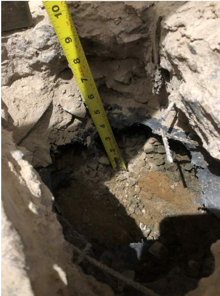
Photograph 13 – Observation hole cut through concrete slab. No water was observed.
