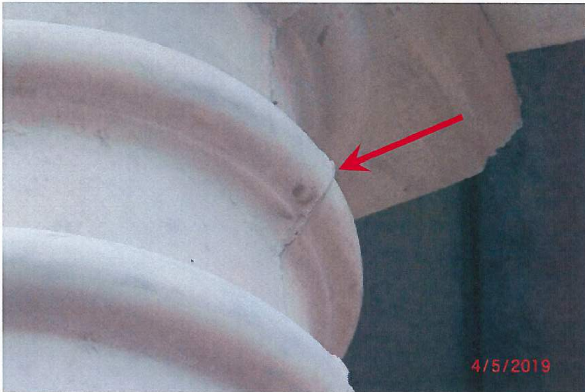
Photograph 5 – Typical seam where halves of column molds met and requires smoothing.
