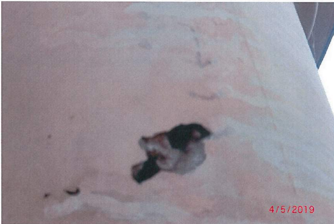
Photograph 4 – Typical bugholes in column surfaces that need to be filled prior or painting/staining.
