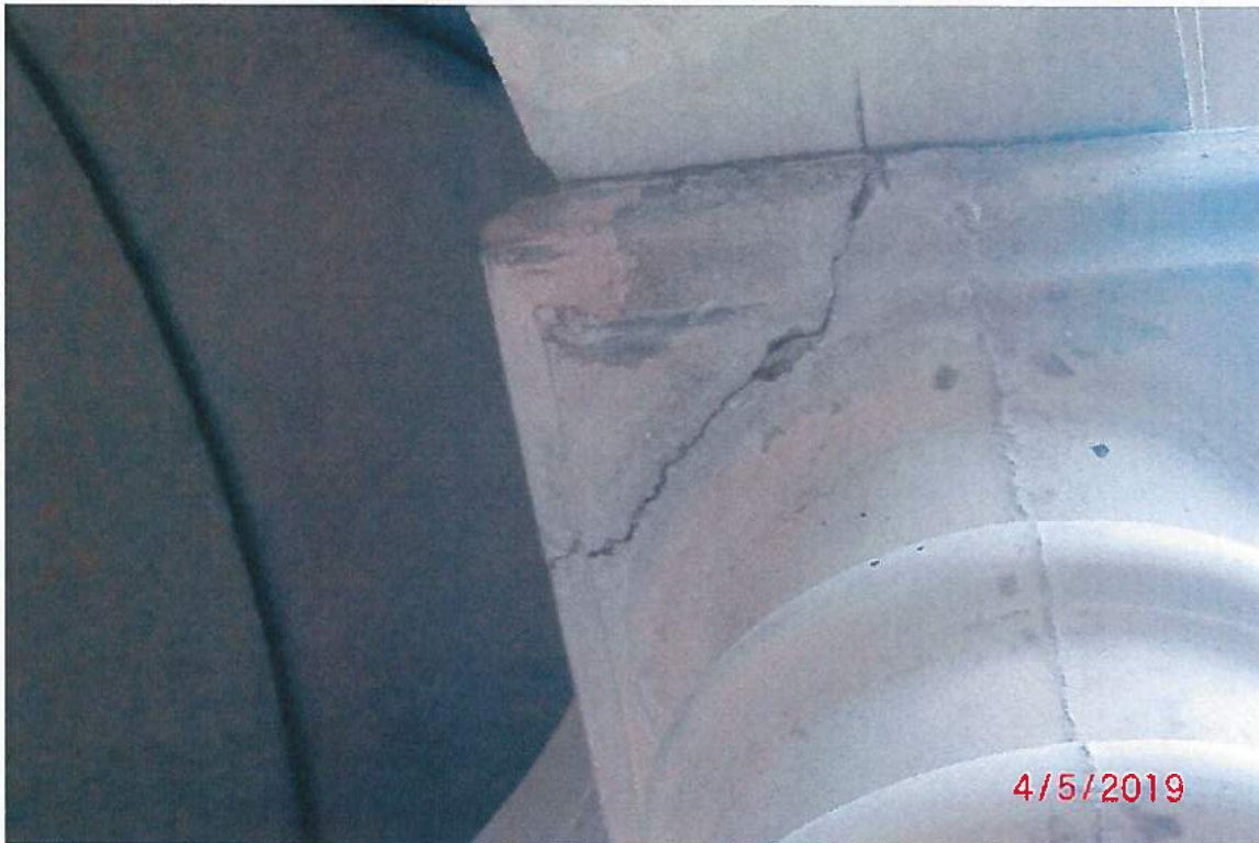
Photograph 7 – Broken section of column capital repaired with epoxy.
