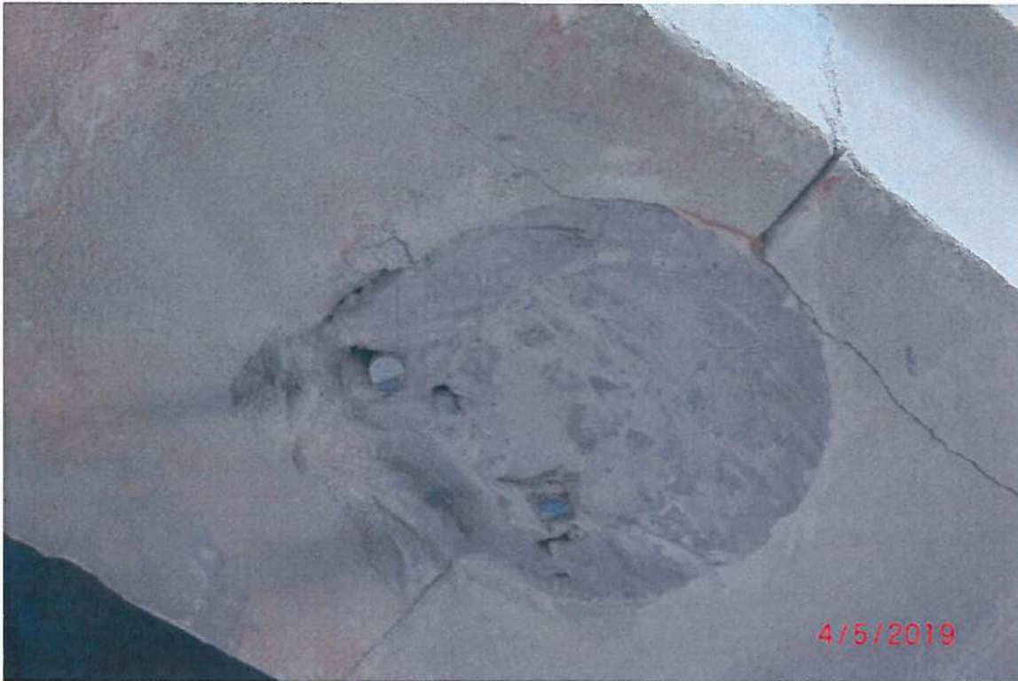
Photograph 9 – Grout filled connection point for original columns with exposed ends of steel bars.
