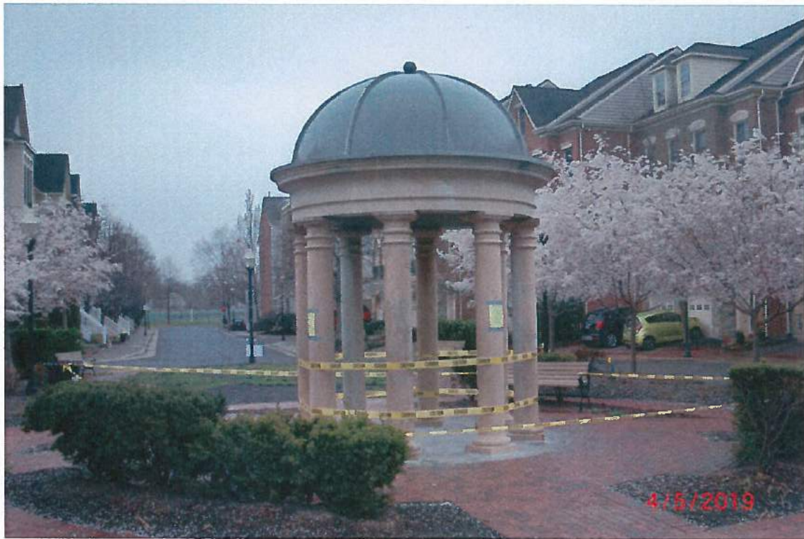
Photograph 1 – Gazebo with new concrete columns and original dome.
