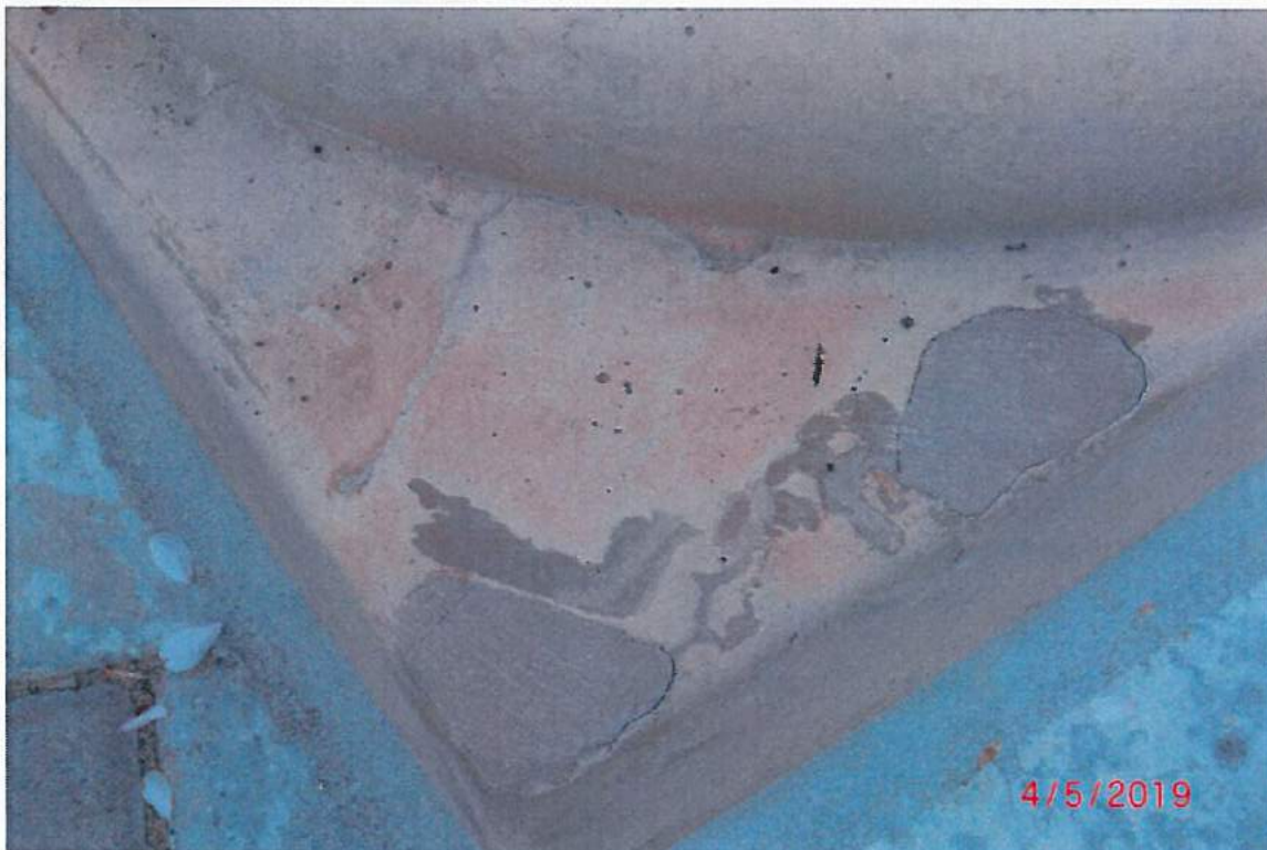
Photograph 6 – Typical factory applied patches that do not match and appear to be separating from the substrate.
