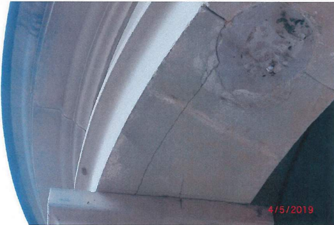
Photograph 10 – Cracks in ring beam at debonded concrete sections.
