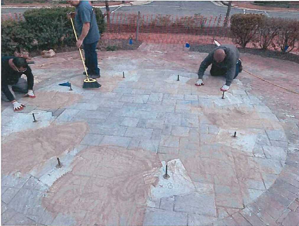
Photograph 3 – Base of the columns with steel bars projecting from the foundation for installation of the new columns. Photograph provided by Soils and Structures, Inc.
