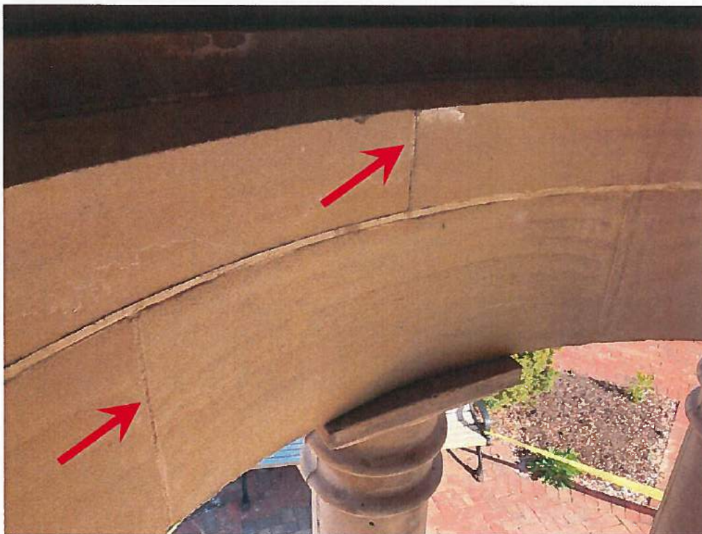
Photograph 8 – Offset joints of ring beam elements.
